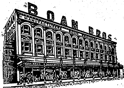
Wellington Street, Frontage
