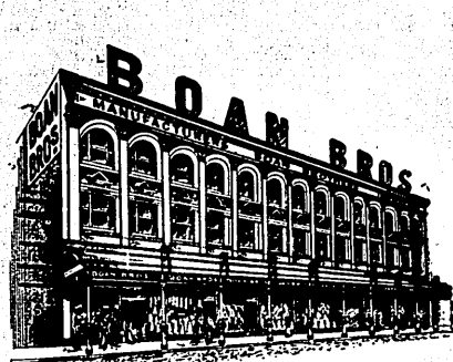
Wellington Street, Frontage
